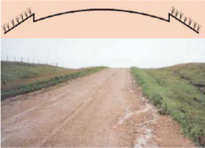
FIGURE 4. Worn blades lead to false shoulders and improper crown.
