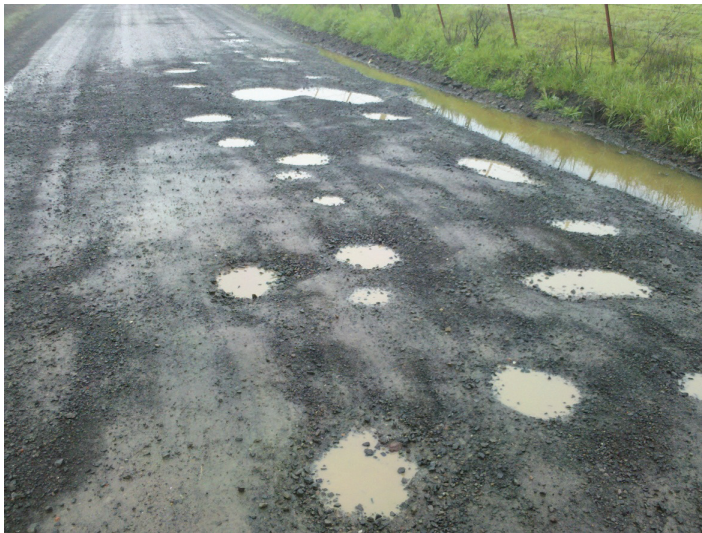
FIGURE 1. This potholed area had 2" of crown and should have been 5".
