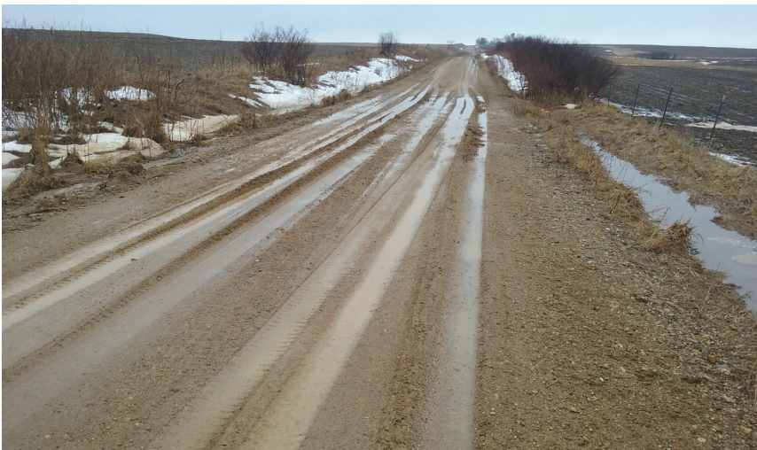
FIGURE 5. Mudhole developing due to lack of crown. Note that the windrow is also holding water on the road. This mudhole is going to get worse.
